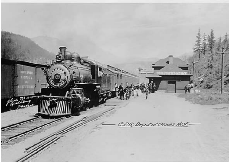
Photo of a CPR train at Crows Nest Station, circa 1920. Could this have been the train that was robbed? Courtesy of Heritage Crowsnest.
