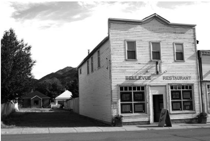
The former Bellevue Café, now with signage Bellevue Restaurant, as it appeared in 2020. The open space to the left is where Office of the Justice of the Peace stood.
